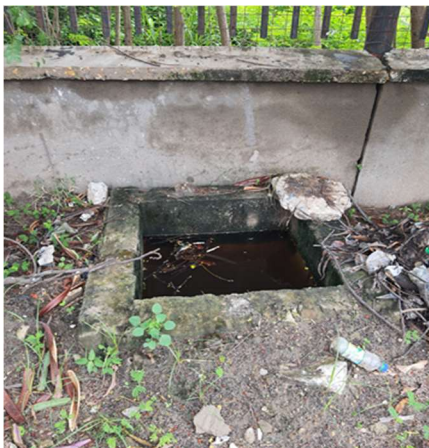
Figure 3.3 Open inspection chamber at the toilet drainage of TOOKU C
